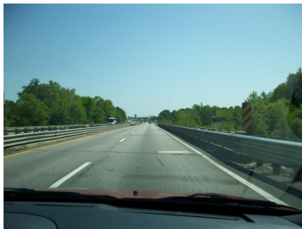
An example of a functionally obsolete bridge.
