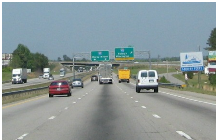
An example of lane and route continuity on I-95.
